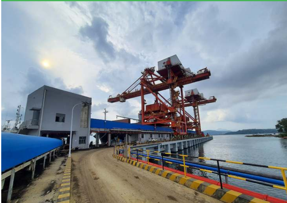
Conveyor Belt in HJF to Replace The Use of Heavy Vehicles
