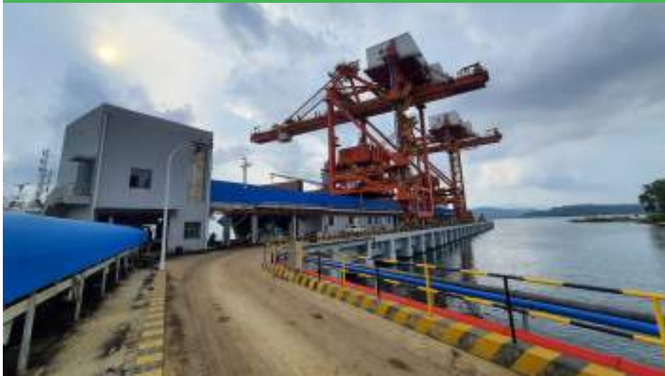
Conveyor Belt in HJF to Replace The Use of Heavy Vehicles
